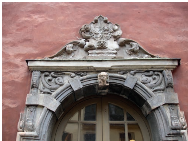
Figure 2 Upper part of the east port of Ryning Palace. The historic paint traces on the stone appear black or grey and are often not investigated prior to maintenance of the façade. (Photo: Anna Henningsson)
