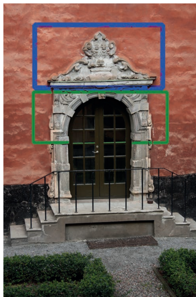
Figure 8. The east portal of Ryning Palace. The blue outline in the picture shows the area where it is extremely difficult to obtain valuable information from the paint traces due to conservation treatments based on acrylic. Therefore, the investigation of the east portal focused on the stone in the central part of the portal (green outline in the figure). (Photo: Anna Henningsson)
